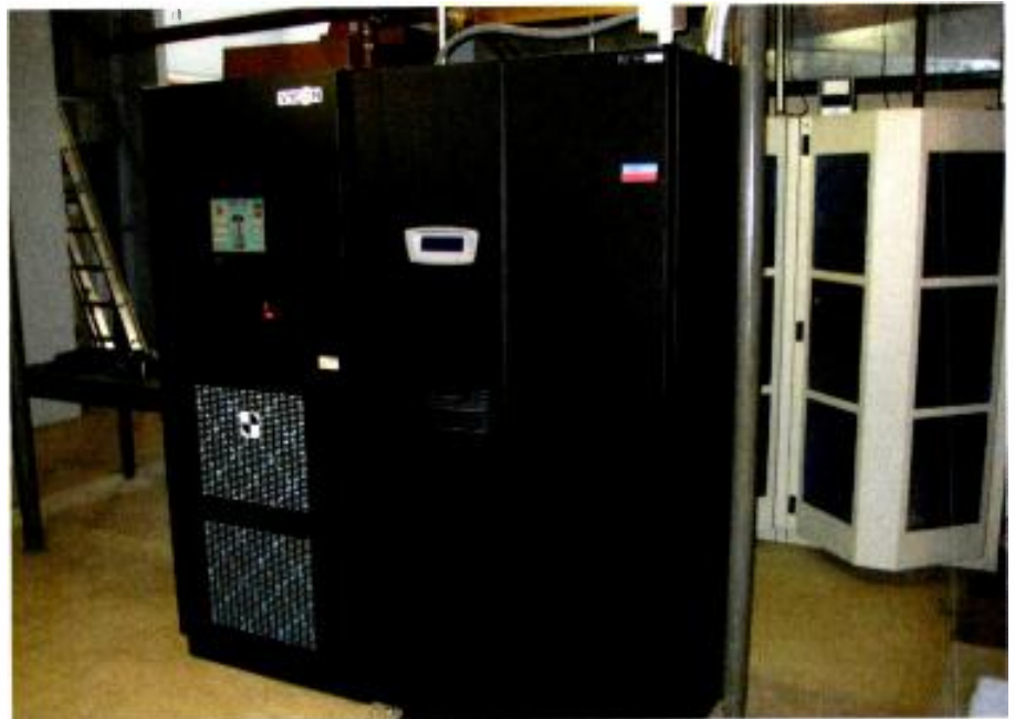
In the event of a power outage, this VYCON VDC flywheel system coupled with a battery-based UPS provides Alabama Public Television with temporary power while the station's generator system fires up.
